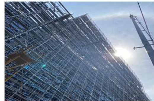
Scaffolding Steel Pipe
